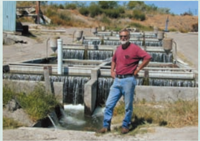
Leo Ray in front of geothermally heated cascading fish raceways. Geothermally heated water accelerates fish growth.
