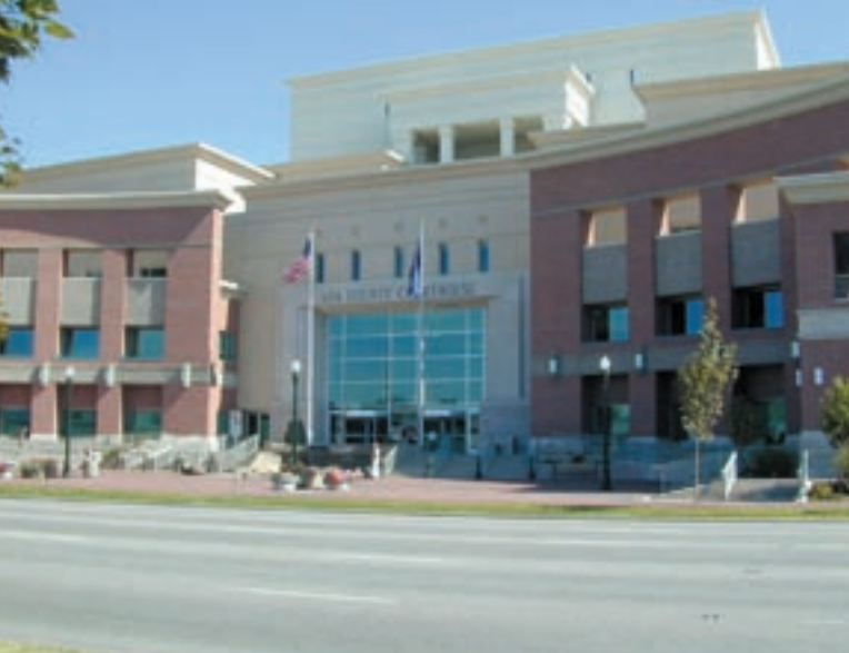
The Ada County Courthouse in Boise, Idaho, uses the city geothermal district-heating system. PIX13078 NREL
